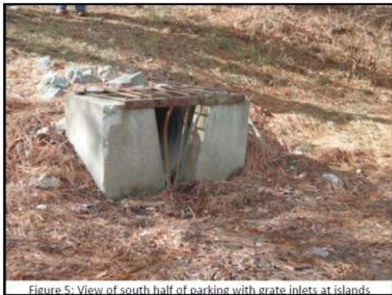
Figure 5: View of south half of parking with grate inlets at islands
