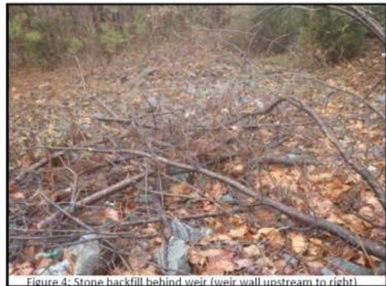
Figure 4: Stone backfill behind weir (weir wall upstream to right)
