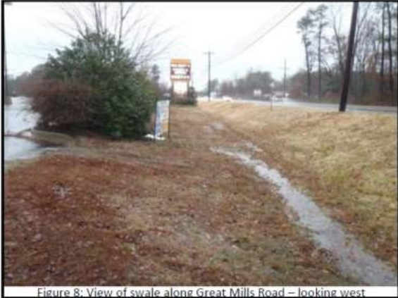
Figure 8: View of swale along Great Mills Road – looking west
