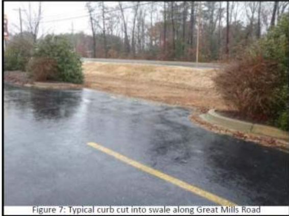
Figure 7: Typical curb cut into swale along Great Mills Road
