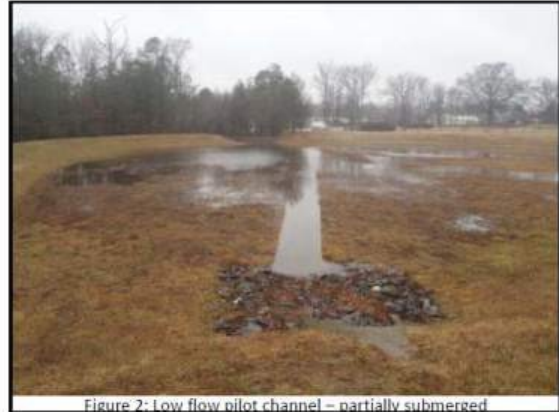
Figure 2: Low flow pilot channel – partially submerged
