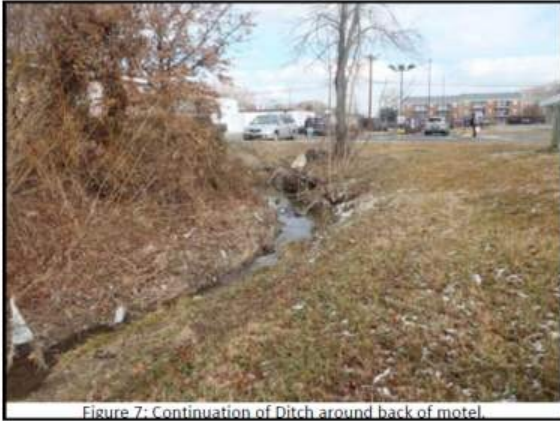
Figure 7: Continuation of Ditch around back of motel.
