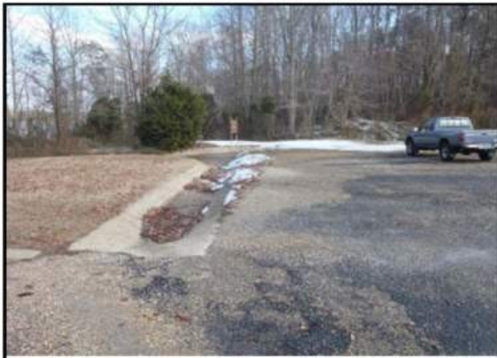
Figure 3: Drainage channel at bottom of parking area – looking east
