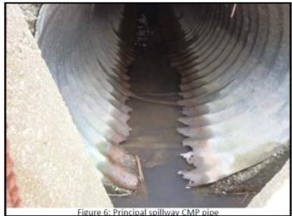
Figure 6: Principal spillway CMP pipe
