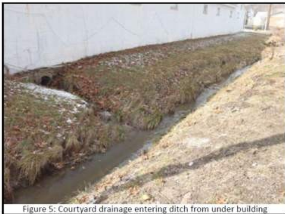
Figure 5: Courtyard drainage entering ditch from under building
