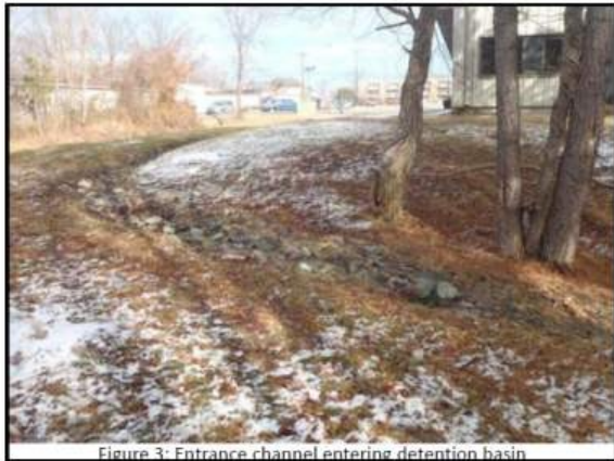
Figure 3: Entrance channel entering detention basin
