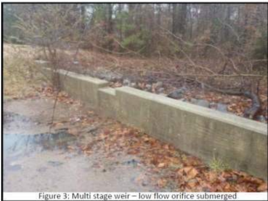
Figure 3: Multi stage weir – low flow orifice submerged
