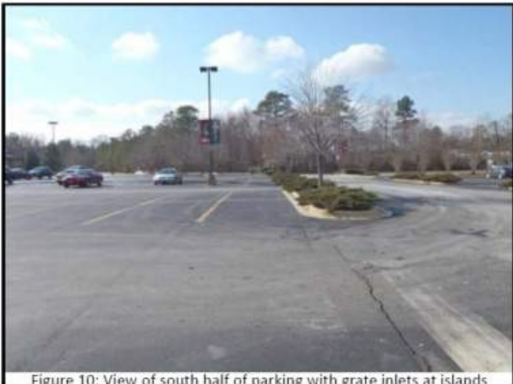
Figure 10: View of south half of parking with grate inlets at islands
